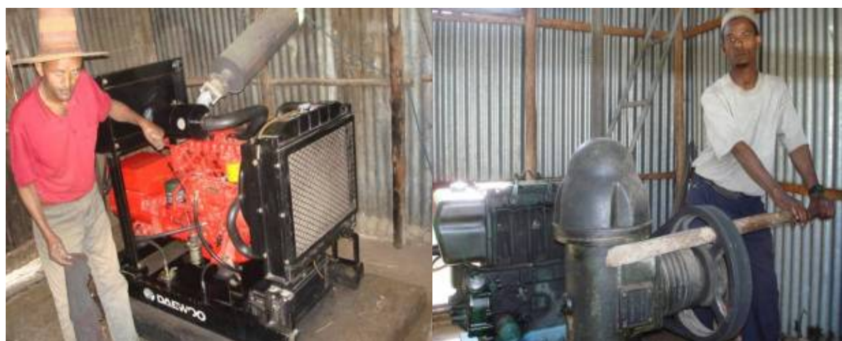
Figure 4.9: Generators of submersible (First Meqala) and mono (Choroqo) pumps
